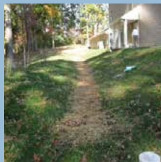
Open Drainage Swale
